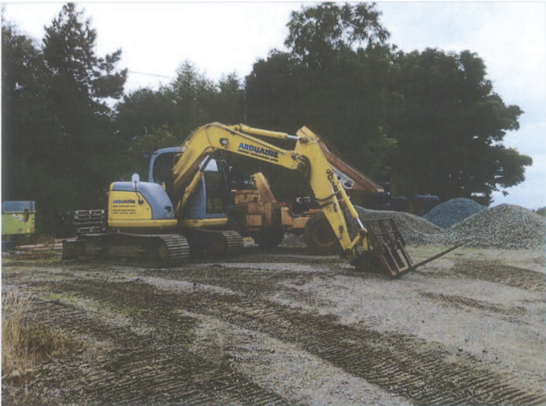
Image 08: Plant, equipment and materials storage area east
